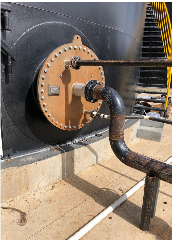
Figure 2. Suction heater installed in a heavy crude oil storage tank. The heating medium is steam with a centre outlet for pumping out warm heavy crude.
